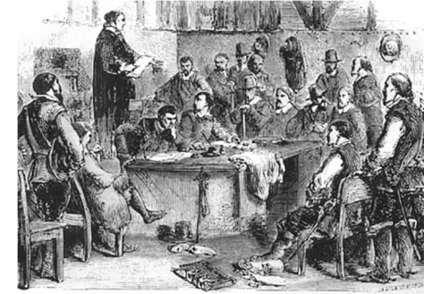
The House of Burgesses, 1619
